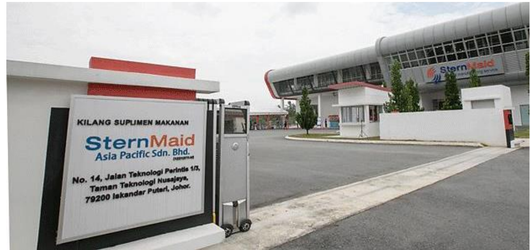
Nusajaya Techpark Facility 2, Johor
