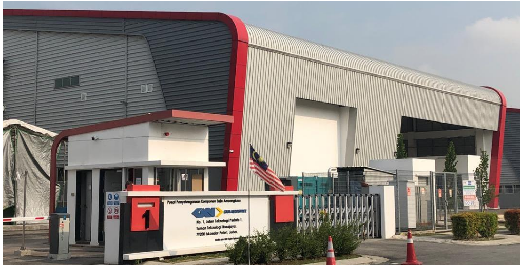
Nusajaya Techpark Facility 1, Johor
